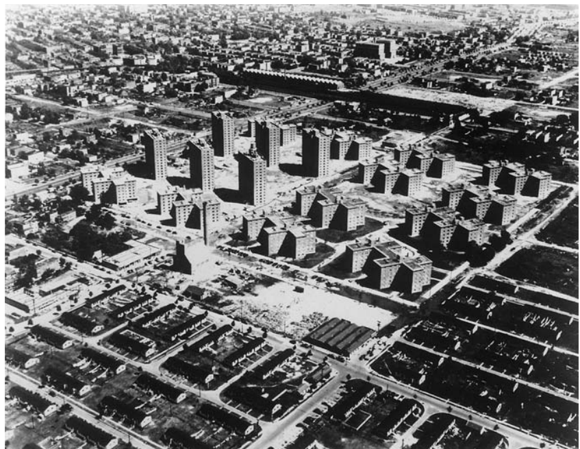
An aerial photograph of Boulevard Houses, a low-income housing project in Brooklyn, illustrates how public housing concentrated poor Americans in structures separated from surrounding neighborhoods.
