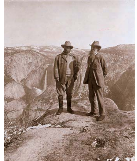
Theodore Roosevelt and the conservationist John Muir at Glacier Point, Yosemite Valley, California, in 1906. Yosemite was set aside as a national park in 1890.
